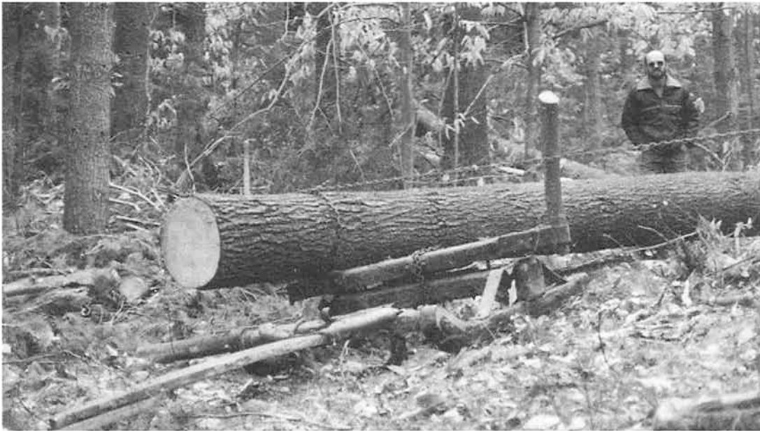
Using cattle to roll on 50' ridge pole, note: butt extends forward over the pole
