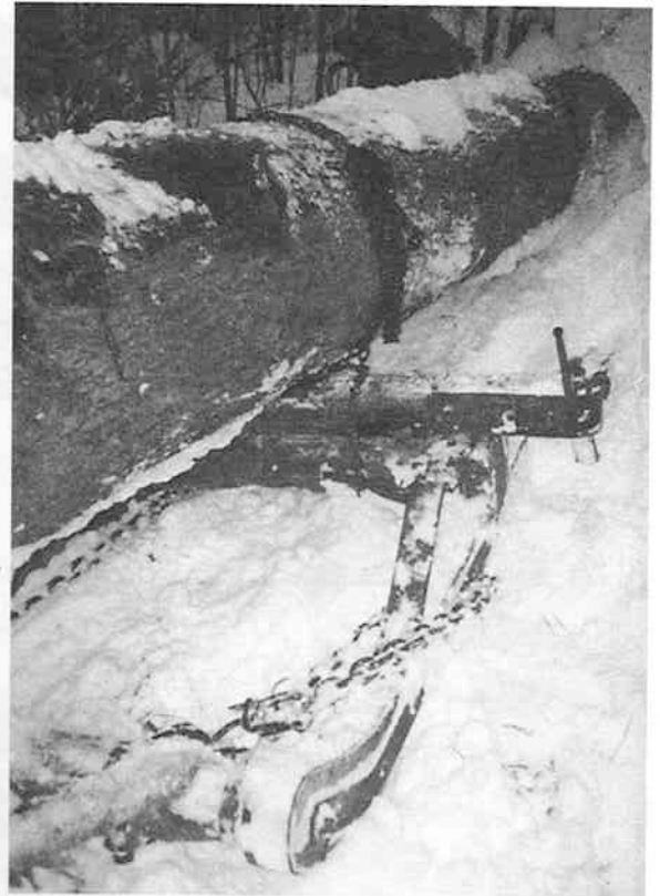
Large white pine log on sled with bridle chain in use, showing finger and ring clasp.
