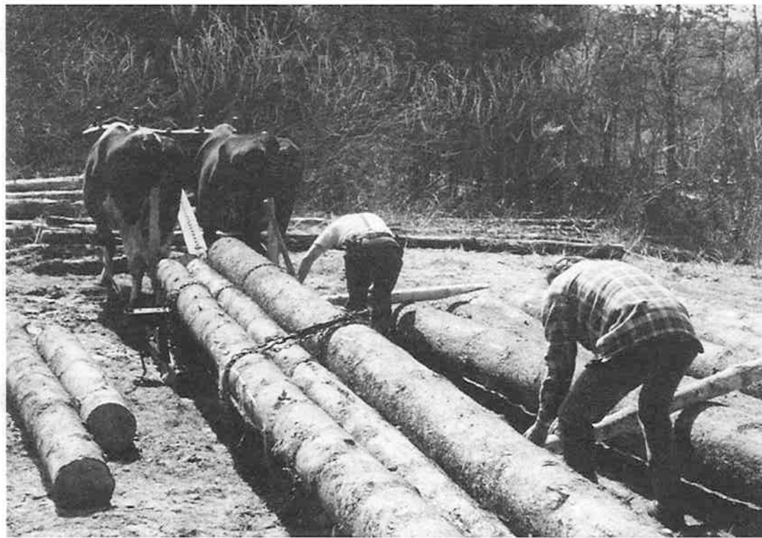
Unloading 34' cabin logs.
